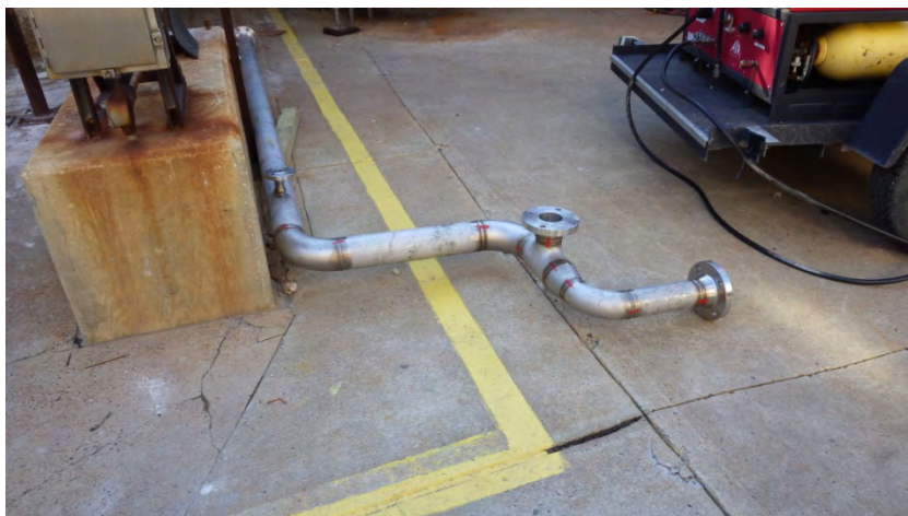
FIGURE 2. 20-foot replacement piping (Source: CSB).
