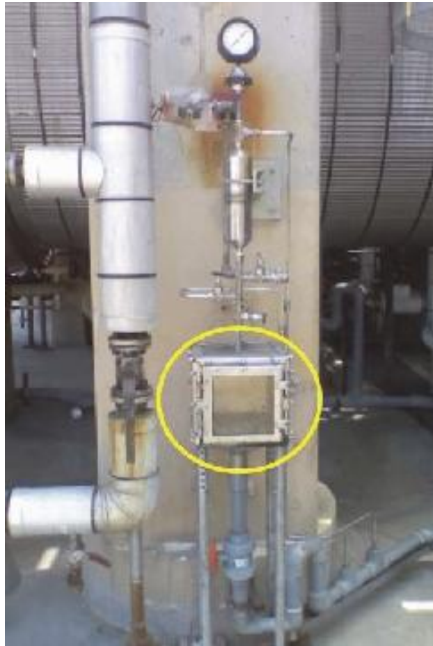
Figure 9. Photo of the sulfuric acid sample station at the Tesoro Los Angeles refinery. This sample system includes an enclosure at the sample point to protect operators from potential acid spray.
