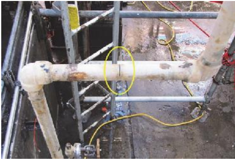
Figure 13. Photo of piping involved with the March 10, 2014 incident. The yellow oval shows the cut the workers made using a band saw that resulted in the acid release. Figure 14 also shows the location of this piping.
