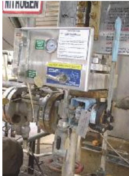
Figure 8. Photo showing one of the upgraded sample stations that Tesoro installed to reduce operator exposure to acid during sampling. Tesoro never resolved the reliability issues with these sample stations and the sample stations were taken out of service. As a result, they were not in use at the time of the February 12, 2014 incident.
