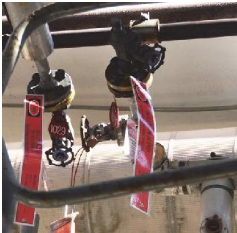
Figure 19. Photo of post-incident isolation of liquid butane supply piping to alkylation reactor. This photo shows the same piping shown in the right photo of Figure 18. Two days after the March incident, Tesoro modified the liquid butane isolation to match the API recommend practice, Tesoro’s corporate standards requirement, and Tesoro Martinez procedure recommendations by disconnecting and installing isolation flanges on each end of the isolated piping.
