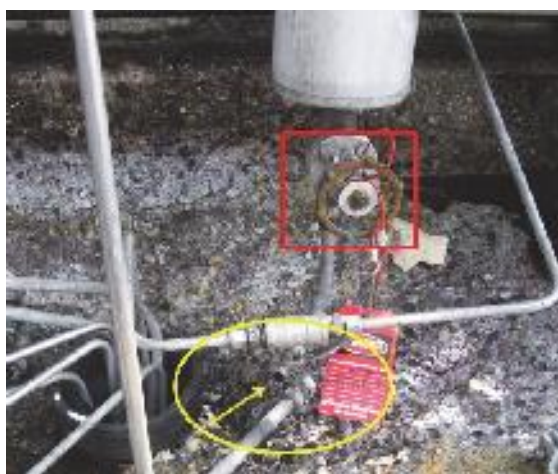
Figure 2. Photo showing the tubing that separated (yellow oval) after the valve (red square) was opened in order to return the sample system back to service following maintenance. Two workers were injured from this acid release incident on February 12, 2014. This loss of containment from the open-ended tubing released 84,000 pounds of sulfuric acid.
