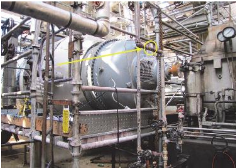
Figure 14. Photo of location of the March 10, 2014 incident. As depicted in Figure 12, two workers were located on this temporary scaffold platform and were cutting the piping (yellow circle) with a portable band saw.
