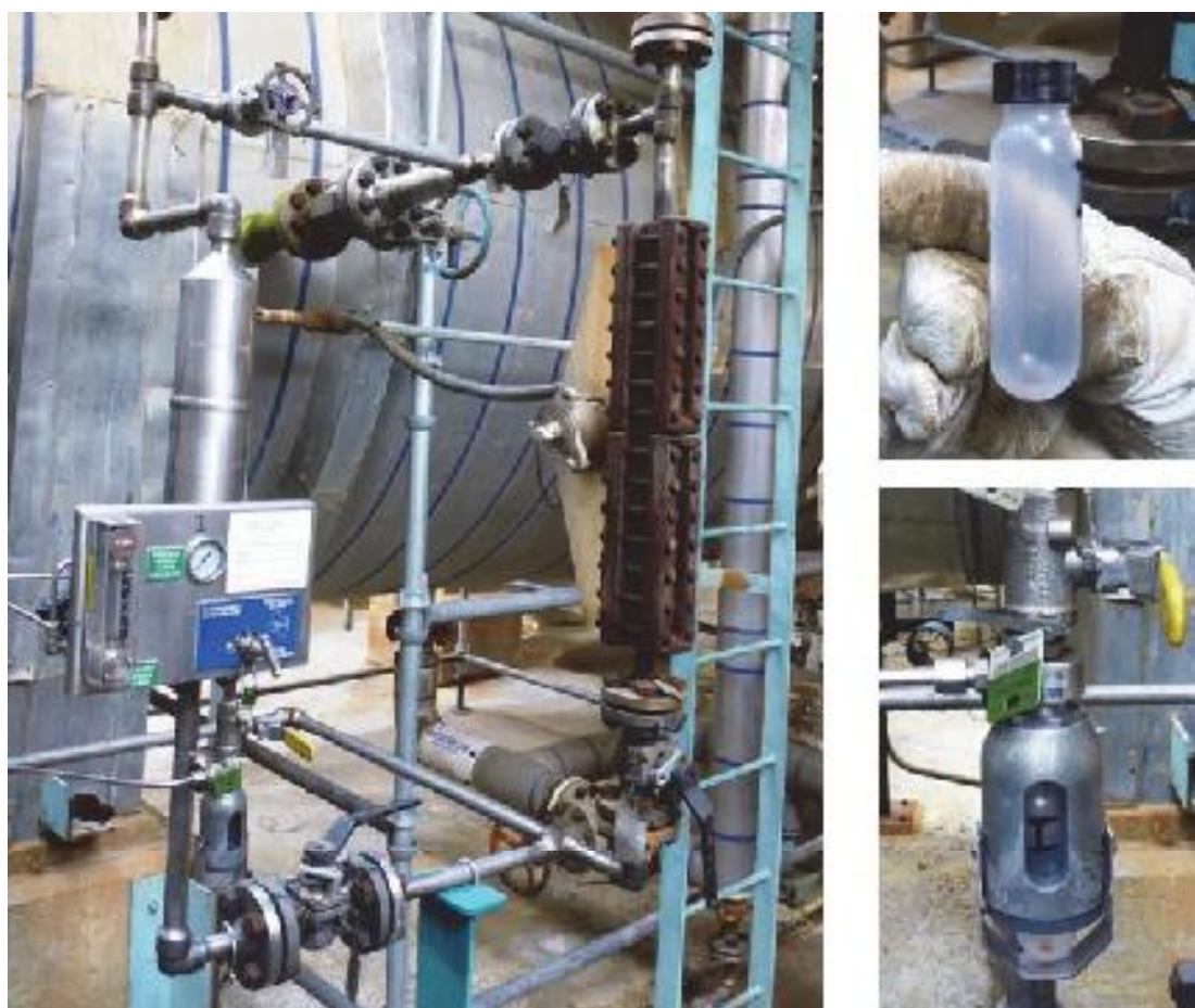
Figure 10. Photo of the sulfuric acid sample station at the Company X refinery. The photo on the left shows a typical sample station used by Company X workers to obtain sulfuric acid samples. The photo on the top right shows a typical sample bottle and the photo on the bottom right shows the sample bottle installed to obtain a sample.
