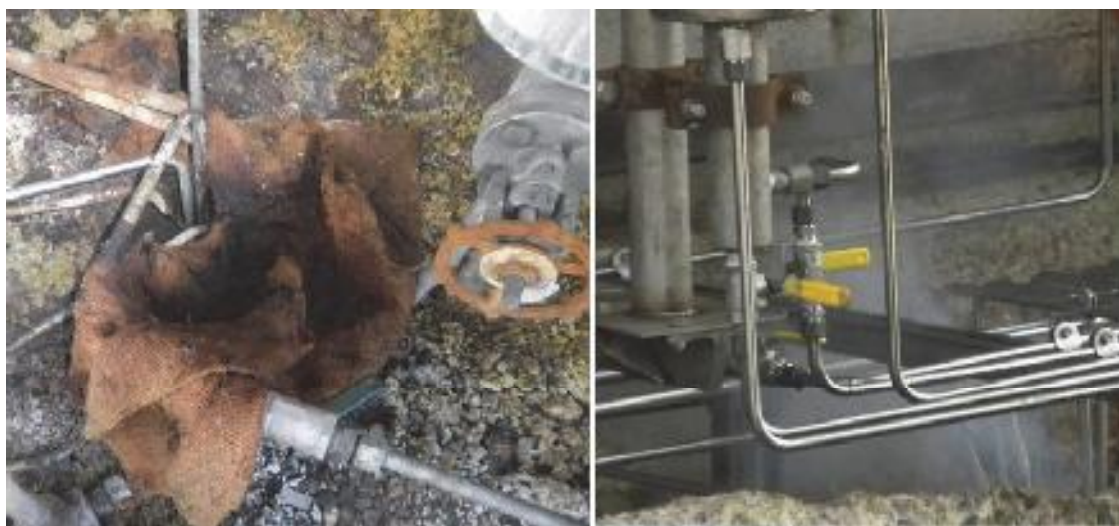
Figure 5. The photo on the left shows a burlap bag covering the process sewer drain at one of the Tesoro Martinez refinery sulfuric acid sample stations. The photo on the right shows the white vapor cloud released from the process sewer drain when Tesoro operators conduct the procedure to sample the sulfuric acid.
