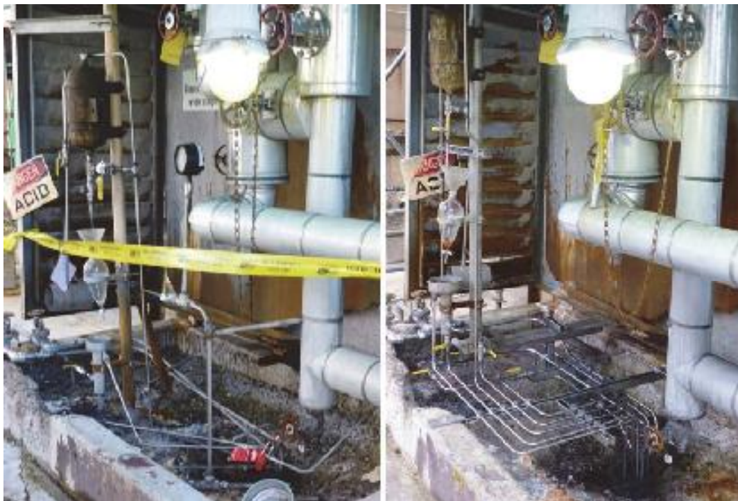
Figure 3. Photo showing the sulfuric acid sampling station at the Tesoro Martinez refinery. The photo on the left shows the sample station just after the February 12, 2014 incident and the photo on the right shows the sample station after repairs were made and the alkylation unit was again operating. Workers informed the CSB that the concrete containment area, clearly visible in the photos above, had badly deteriorated from routine exposure to sulfuric acid.
