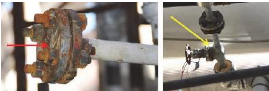
Figure 18. Photo of piping isolation at time of March 10, 2014 incident. The photo on the left shows the piping isolation on the reactor side. A blind flange (red arrow) was installed in December 2013 when the piping was disconnected from the alkylation reactor. The photo on the right (yellow arrow) shows the single valve used to isolate butane from the piping workers were cutting.
