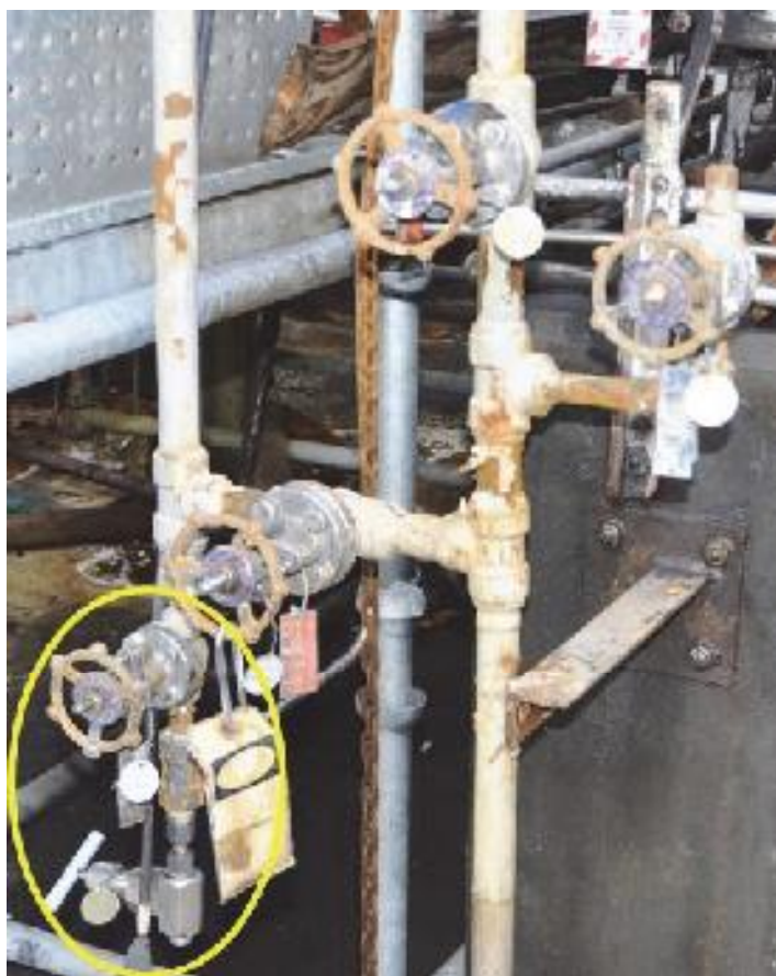
Figure 16. Photo of drain piping and valves. Evaluation of this equipment after the incident identified plugging in these piping components that prevented liquid from freely draining through the open valves.
