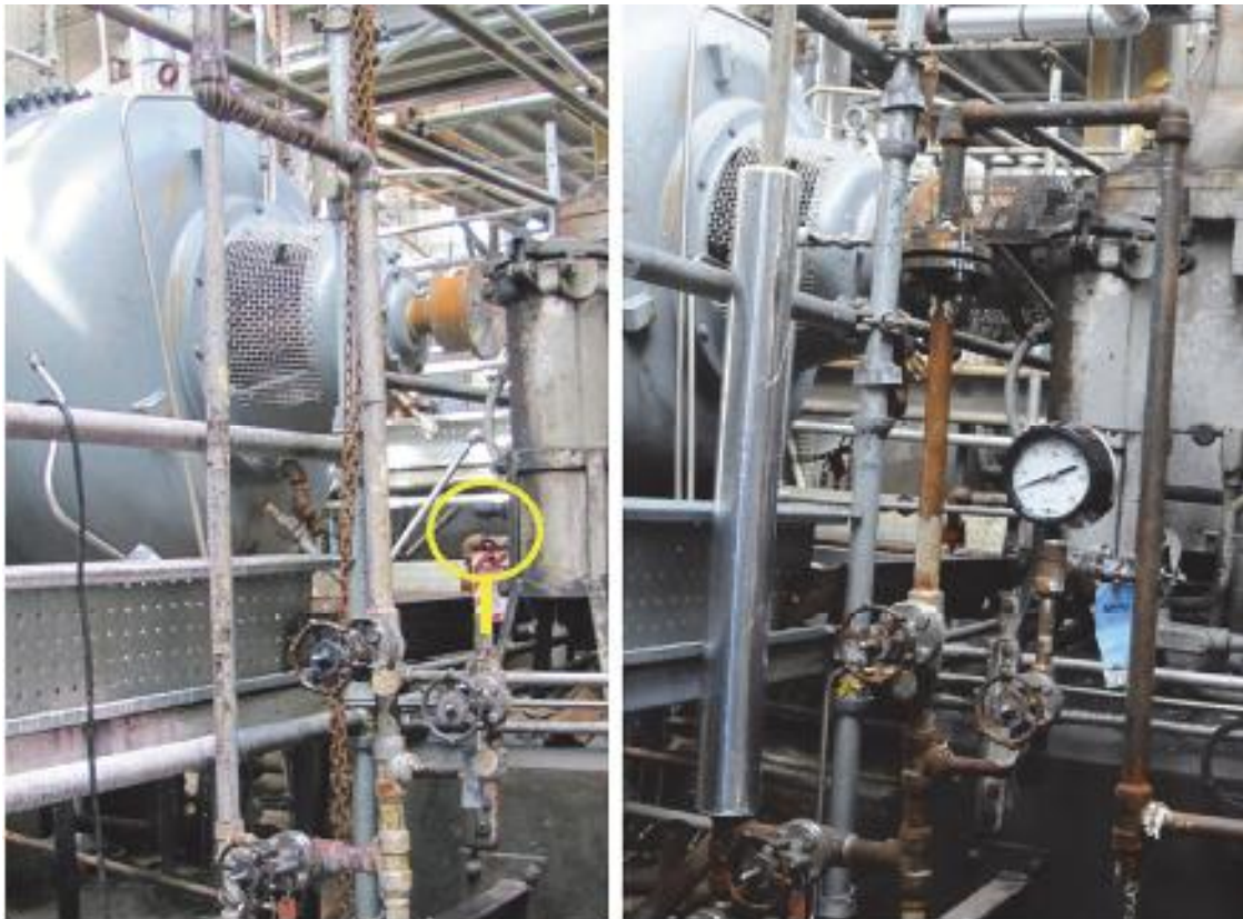
Figure 17. Photo of piping involved with the March 10, 2014 incident (left photo). The photo on the right shows the piping after repairs were made and the pressure indicator was reinstalled. Note the yellow circle in the photo on the left that shows the location where a pressure indicator was supposed to be located, but had been removed. Had this pressure indicator been available it could have alerted workers that dangerous pressure remained in the piping system.
