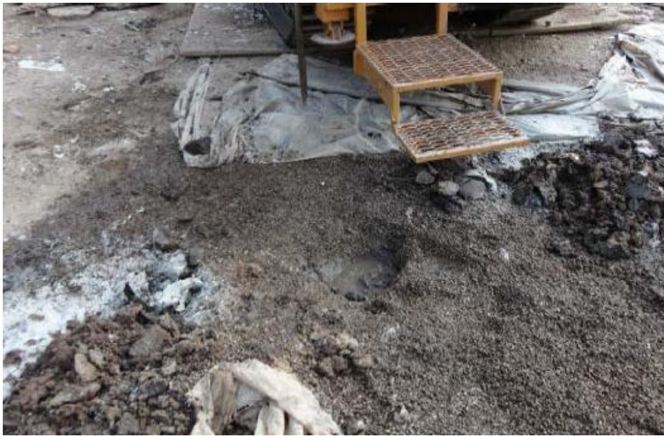
Figure 20. Gravel base under tank 396 and other MCHM tanks. (Source: Terracon)
